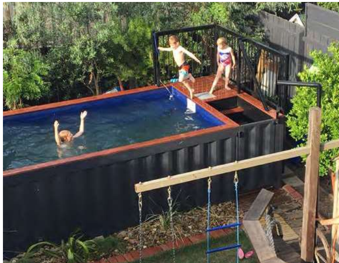
⬆ The above-ground recycled shipping container pool is, of course, one of the kids' favourite features of the house. Supplied as a self-contained unit complete with access steps, pump and filter, it was chosen for the minimal groundwork required to install it, avoiding the unknown cost of excavation needed for a conventional pool. Homeowners' photo.
